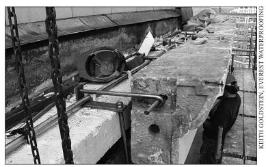
**RESTORATION UNDERWAY** on a terra cotta cornice. The century old original units were salvaged and are being reattached using stainless steel rods.
