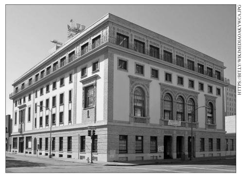
**THE YWCA BUILDING**, built by Julia Morgan, provides an early example of color used on a ceramic façade. It's also a good example of the use of a matte glaze finish.
