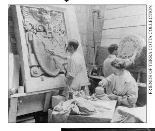
**IN 1915**, artists at the O. W. Ketcham Terra Cotta Works modeling shop sculpted the clay master copies of each piece. Plaster working molds were made from these, with allowances for clay shrinkage.
