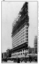
A CURTAIN WALL of terra cotta is being fastened to the steel structure of New York's Flatiron Building, 1902.
