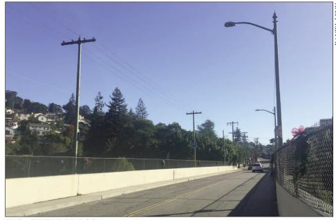
THE LEIMERT BRIDGE boasts trolley poles converted into lighting standards.
